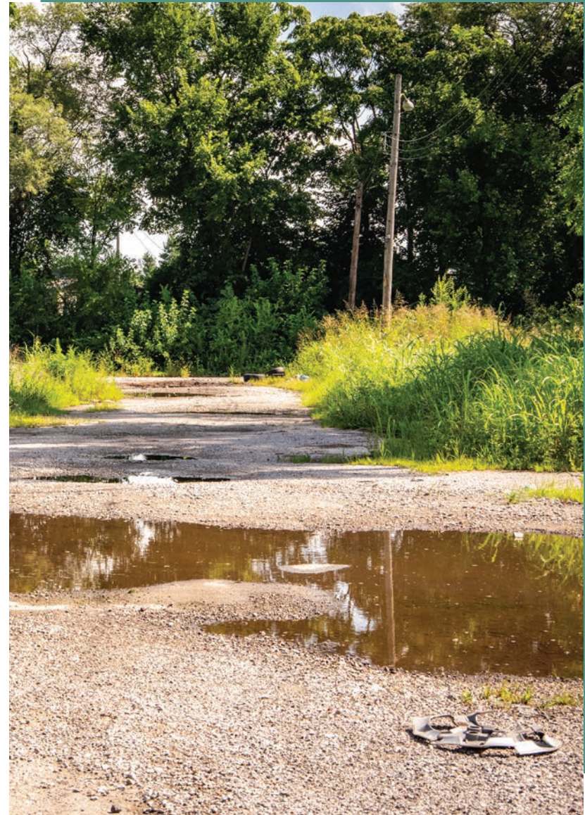
Figure 10.22 A street flooding due to poor drainage.
